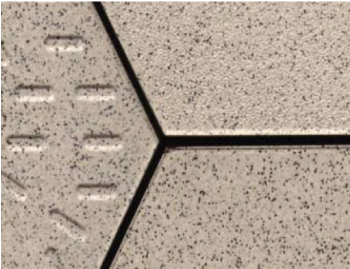
2. Hexagonal, Carolina Clay, fully-vitrified TUFCHM tiles used at BI Chemicals
